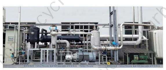
Photo of 800Nm<sup>3</sup>/h Dichloromethane gas recovery equipment on site
