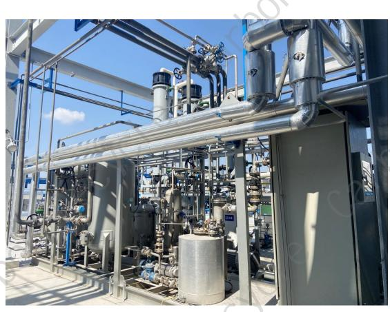
Fig. 7:Photo of 600Nm<sup>3</sup>/h propylene oxide solvent recovery equipment on site
